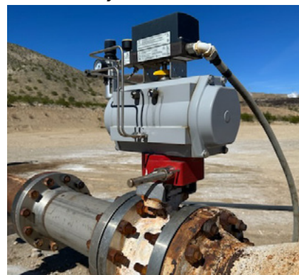
Bray Series 19L segmented ball valve remains in service after 2½ years of continuous duty.
