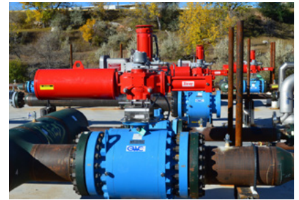
Switching Service — 120VAC powered S98EH spring return actuators mounted on ball valves used on a pipeline manifold.
