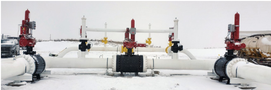
(Above and Right) Line Break Service — 24VDC powered S98EH double acting actuators with stored energy accumulator mounted on ball valves.
