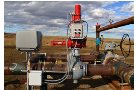
Switching Service — 120VAC powered S98EH spring return actuators mounted on ball valves used on a pipeline manifold.
