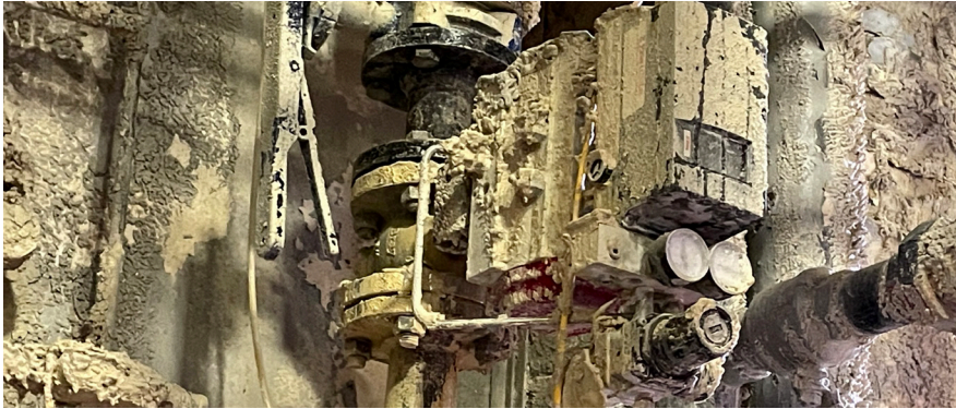
Bray Series 19L control valve package in Milk of lime service.
