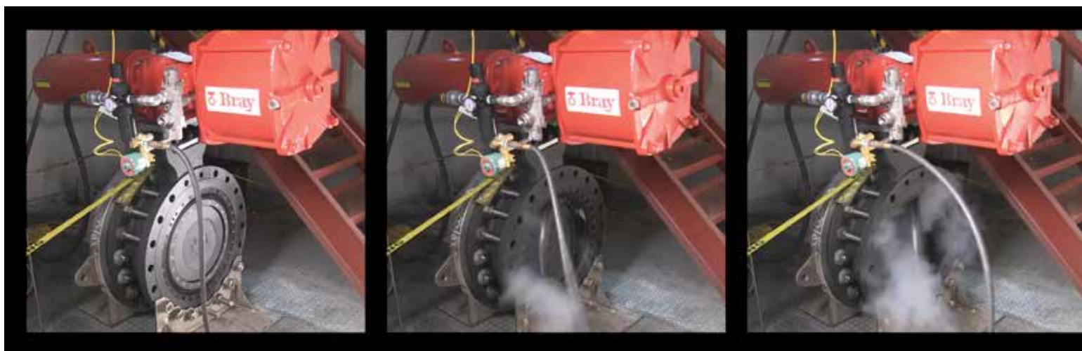
A Bray Tri Lok triple offset valve with Series 98 pneumatic spring return actuator and hydraulic dampener for blowdown service.
